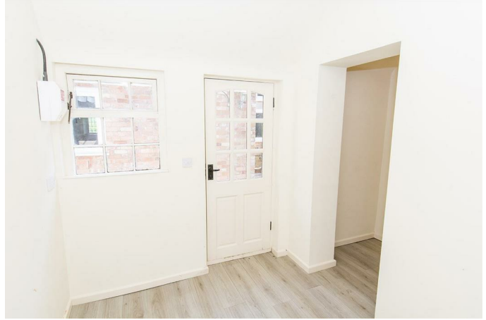
Single-glazed timber entrance door and window. Opening through to store room.
